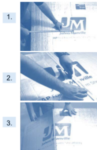
Figure 1. Vented Ceiling – Across Rafters
